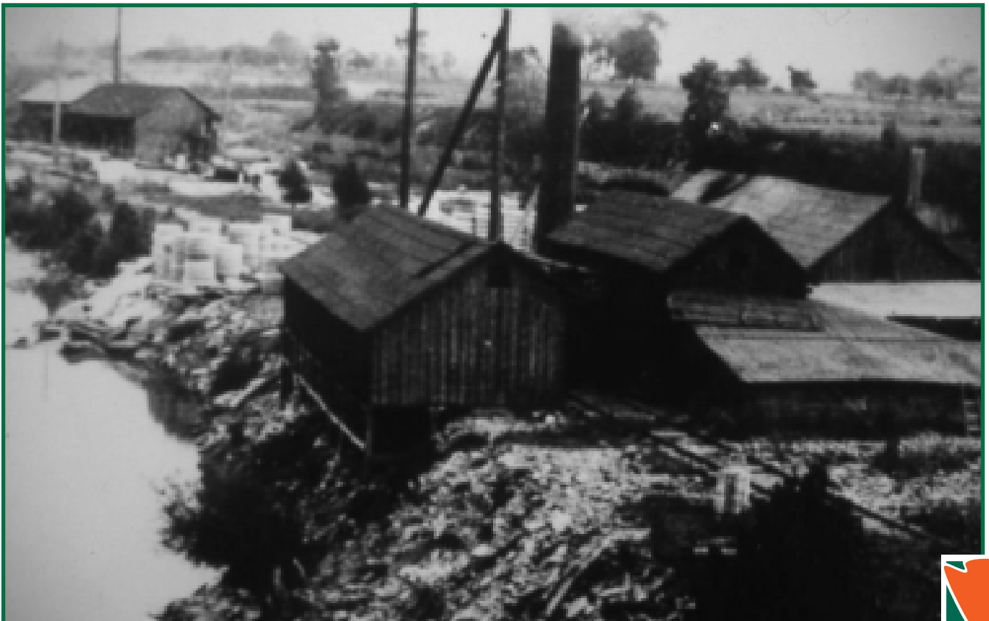
Standing on an old railroad bridge and looking southwest in 1900 would give you a view of these quarry buildings. The two buildings in the upper left corner are the grindstone block saw buildings. The three buildings in the middle were the grindstone lathe buildings.
