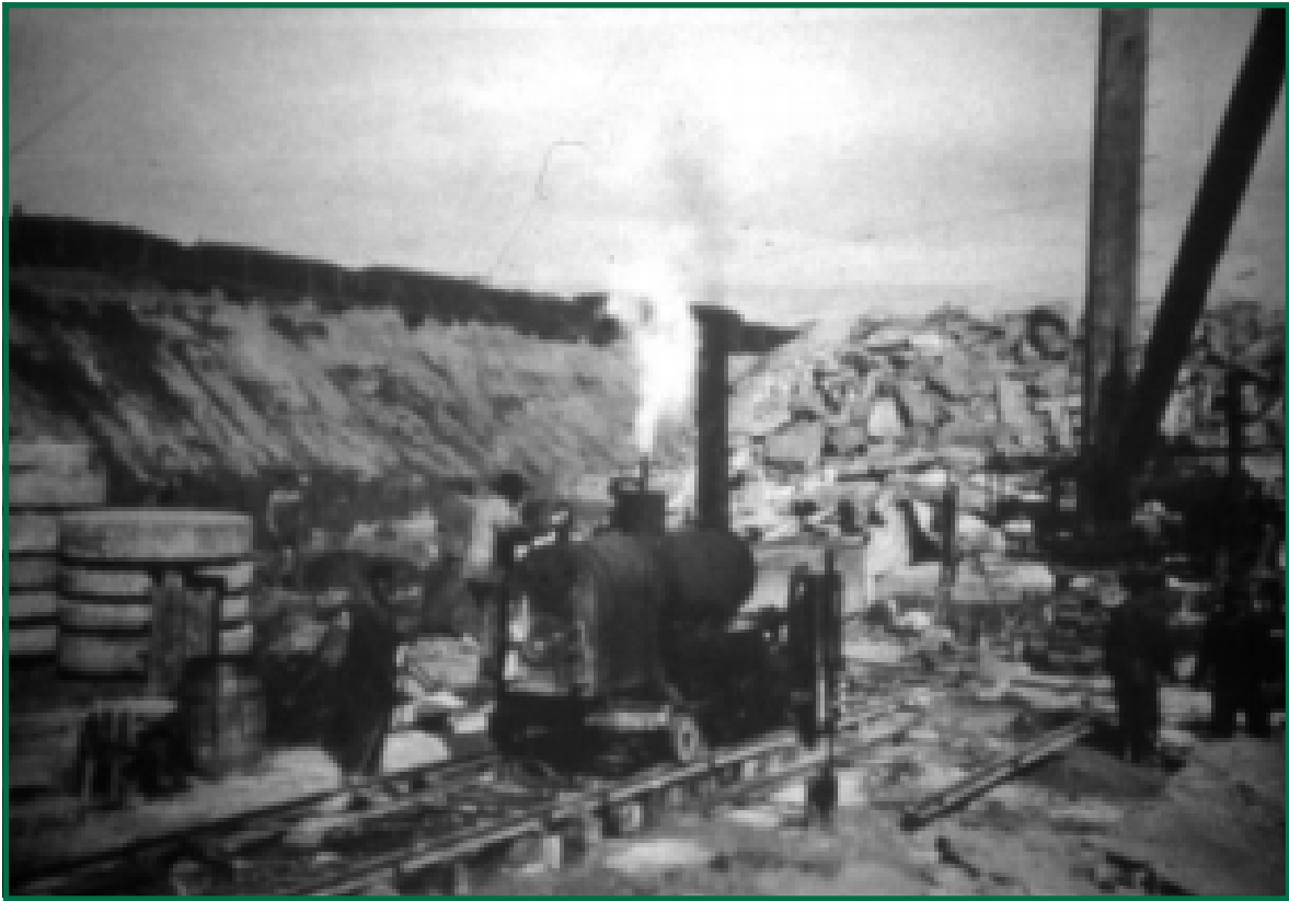
This channeling machine, invented in the 1880s, chiseled into solid stone and created huge blocks. It was also used to cut grindstones directly out of the ground, as seen in this photo.
